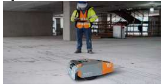
Fig. 3 - Layout with Dusty Robotics
