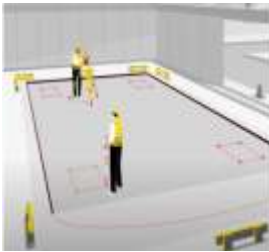
Fig. 2 - Layout with Total Station
