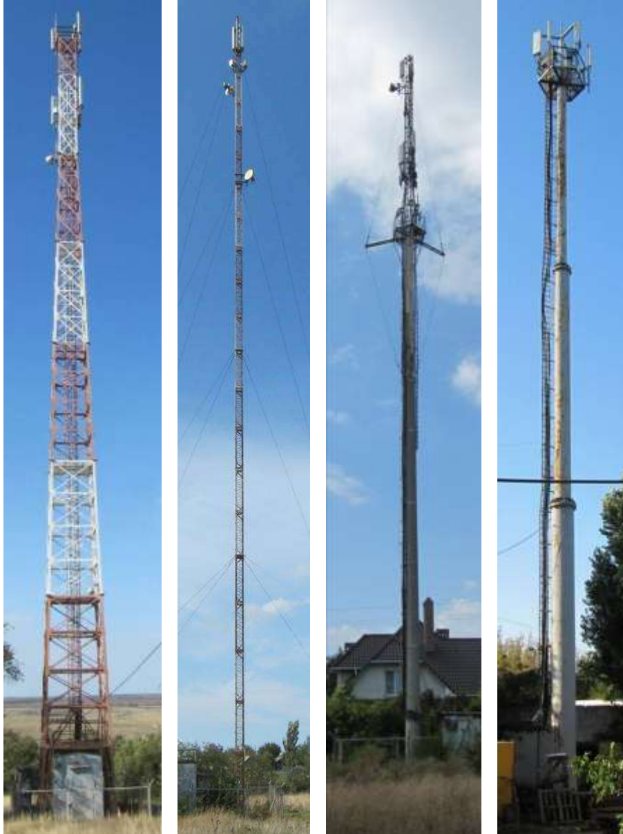
Fig. 1. General view of the most common types of antenna structures
