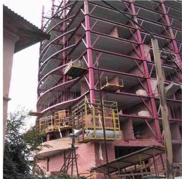
Residential building during construction
