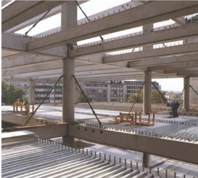
Steel concrete frame multi-storey of industrial building
